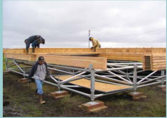
Construction of the Kongiganak FSC
