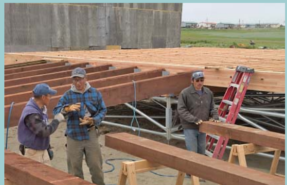
Construction of the Hooper Bay FSC
