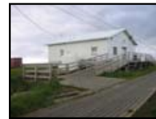
Kipnuk Halibut Plant
